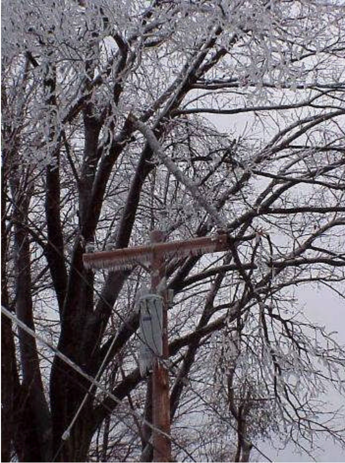
Figure 1 Branch failure due to ice loading is a major cause of interruptions during ice storms.
